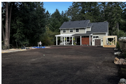
Before: Prepped & Rolled
